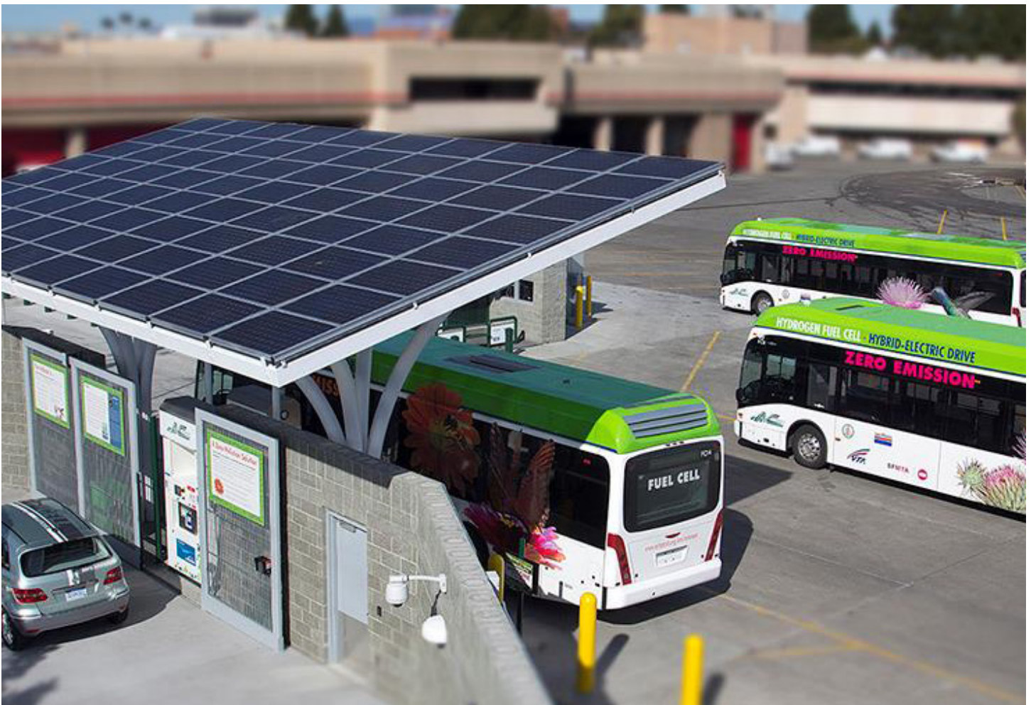
Figure 3: Hydrogen refueling station at AC Transit, California
