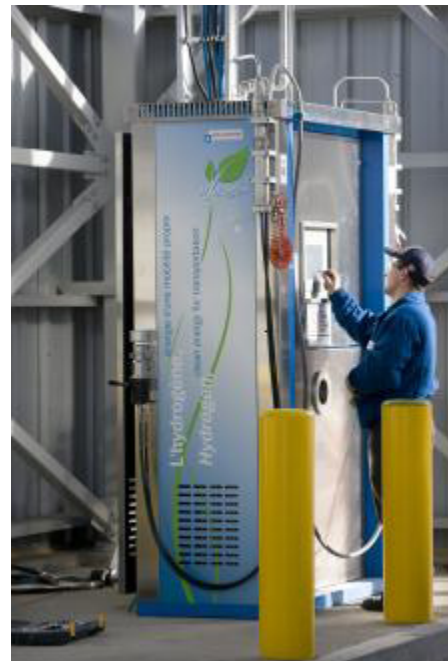
Figure 2: Hydrogen Dispenser by Air Liquide
