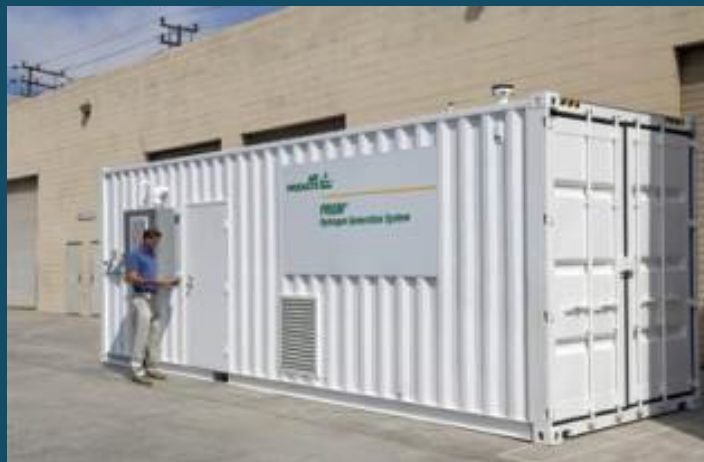
Figure 11: Air Products PRISM On-Site Hydrogen Generation System
