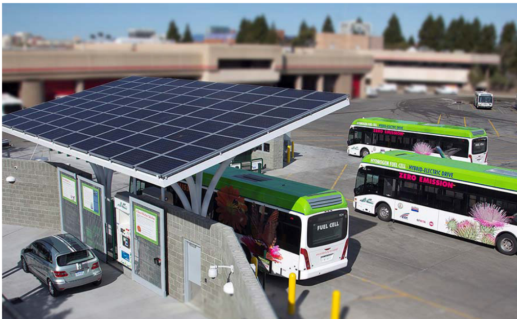
Figure 6: AC Transit / Linde Emeryville, CA Hydrogen Refueling Station
