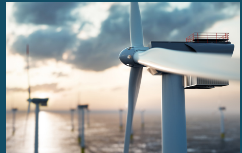
1.2MW (DC) offshore peak shaving power generation at Hollandse Kust Noord offshore wind project
